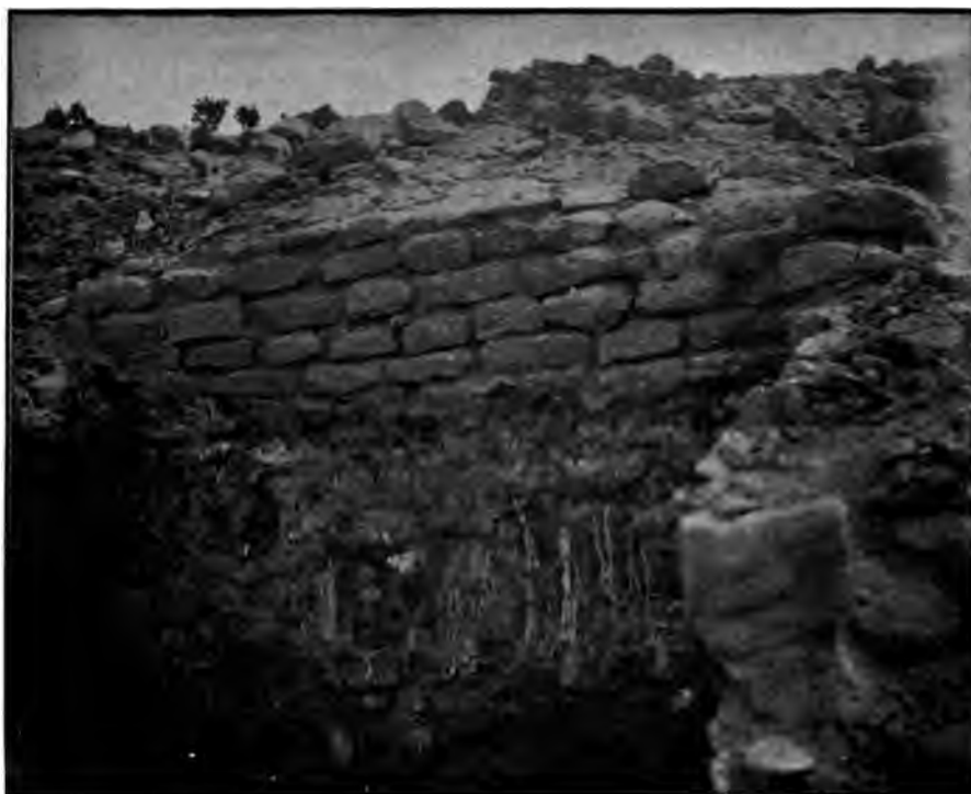
FIG. 256—Structure of house wall of Awatobi
